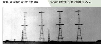
Fig. 1: Historical photograph (hence quality!) showing the antenna systems of a typical East Coast Chain Home (CH) station. The four towers in the foreground carry the transmitting antennas and those in the background, the receiving antennas (see text).
